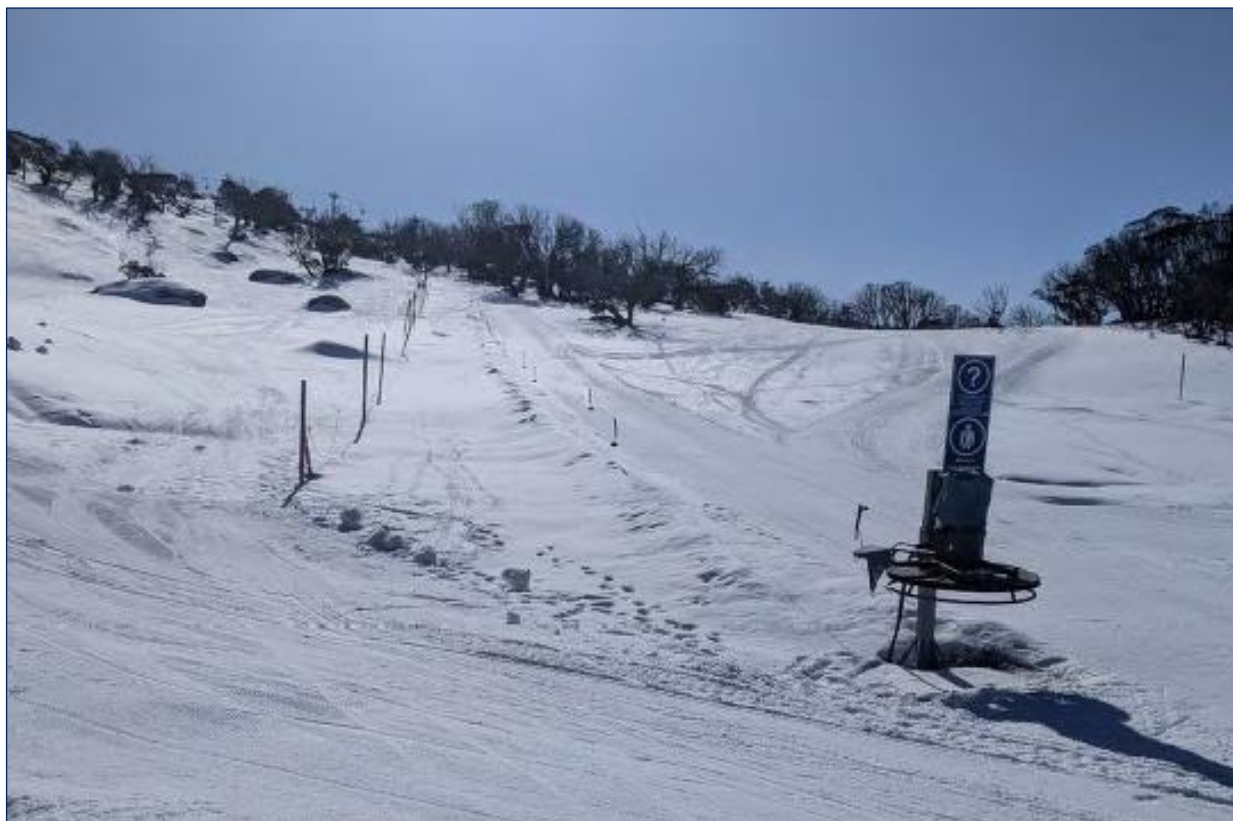
Figure 2 | View of existing rope tow during winter (Source: Applicant's documentation)
